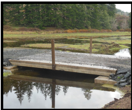
Collapsing culvert replaced with concrete slab bridge at a livestock crossing
