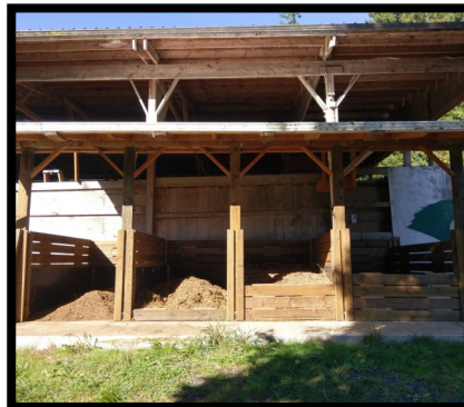
Four-bay manure storage and composting facility installed at a local horse boarding operation
