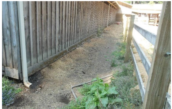
Main Barn, adjacent drainage: AFTER (8-8-2018)
