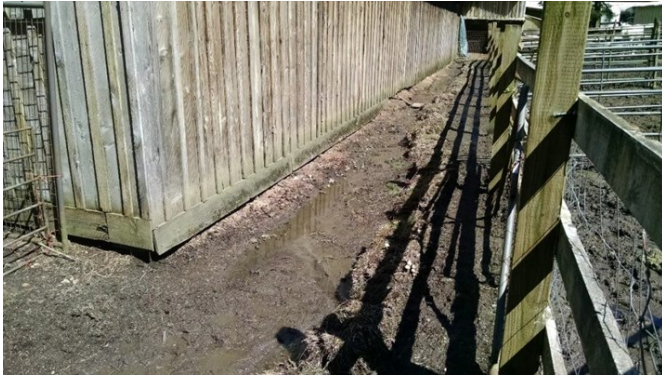
Main Barn, adjacent drainage: BEFORE (6-14-2017)
