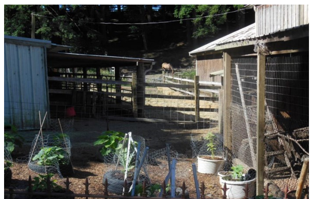
Main Barn, adjacent drainage (facing south). AFTER: Culvert has been installed so that there is no longer any above-ground flow through the stable yard; tree removed and vegetable garden planted (7-3-2018).
