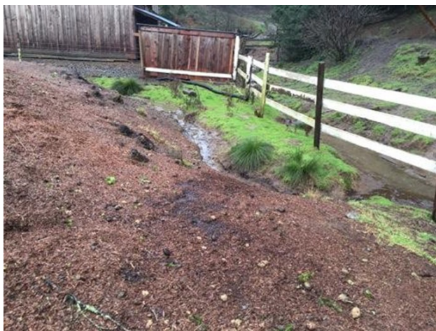
Initial site visit, December 2015 shows highly concentrated manure- runoff flowing directly into the tributary stream
