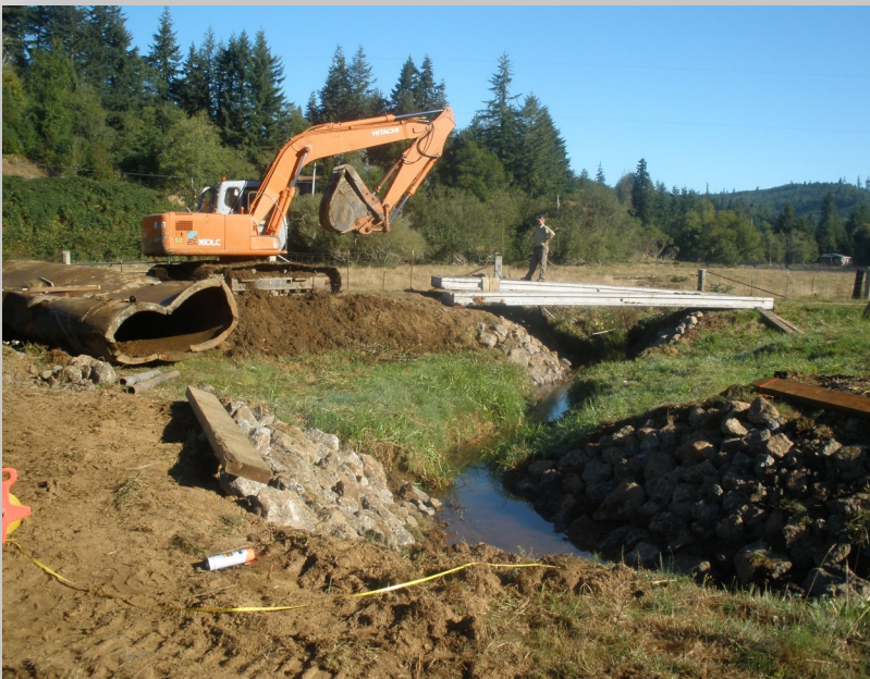
Work completed by Messerle & Sons.
