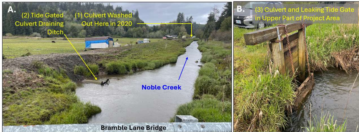
Figure 23. Photos of Current Locations Where Interior Culvert and Tide Gate Improvements are Proposed. (A) View Looking Downstream at Leveed Section of Noble Creek from Bramble Lane Bridge. (B) Photo of Tide Gate and Leaking Culvert in the Upper Part of Project Area
